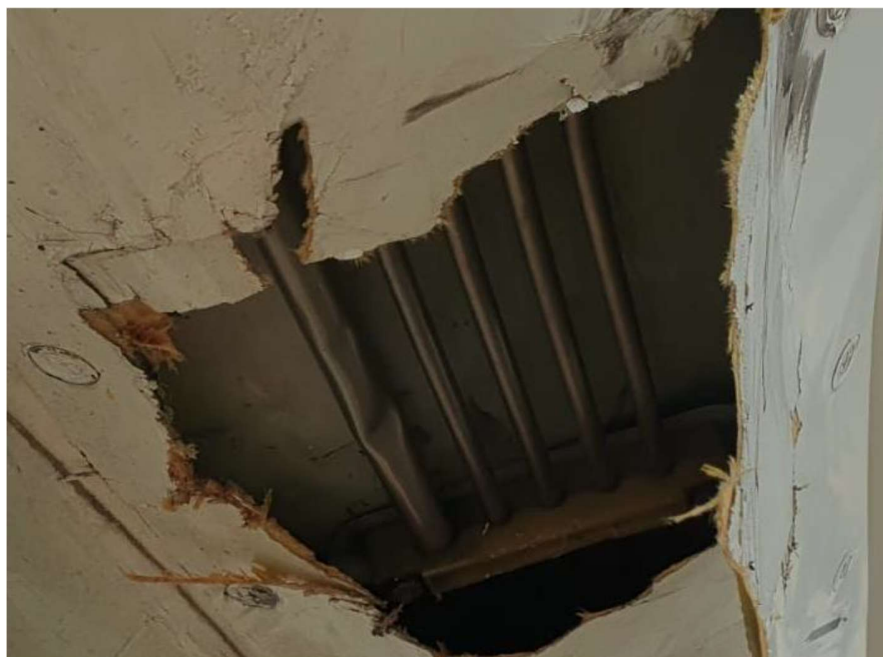
Picture 3 - hydraulic pipe
