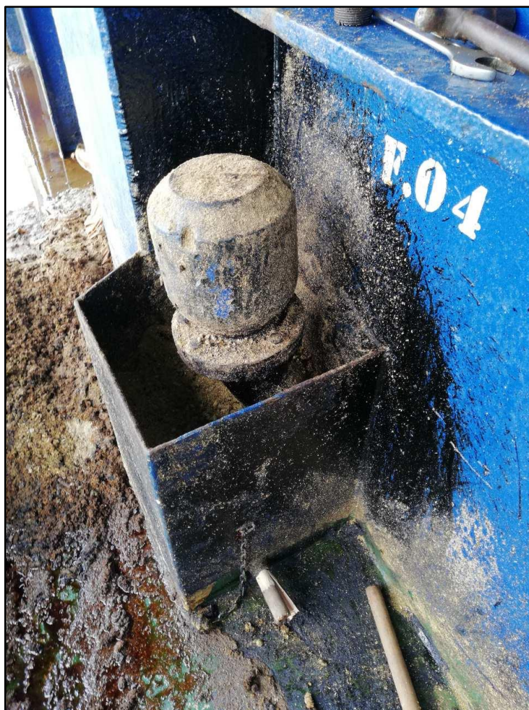
Picture 4 Marine Residual Fuel on the deck and on the vent of the Fuel tank no 4
